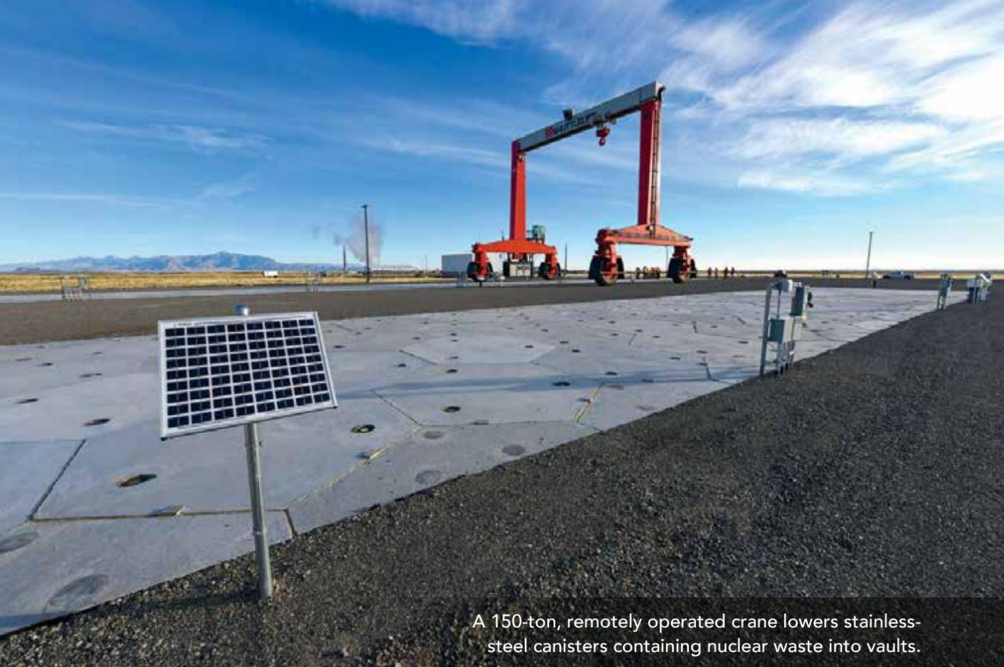
A 150-ton, remotely operated crane lowers stainless-steel canisters containing nuclear waste into vaults.
